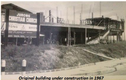
Original building under construction in 1967
